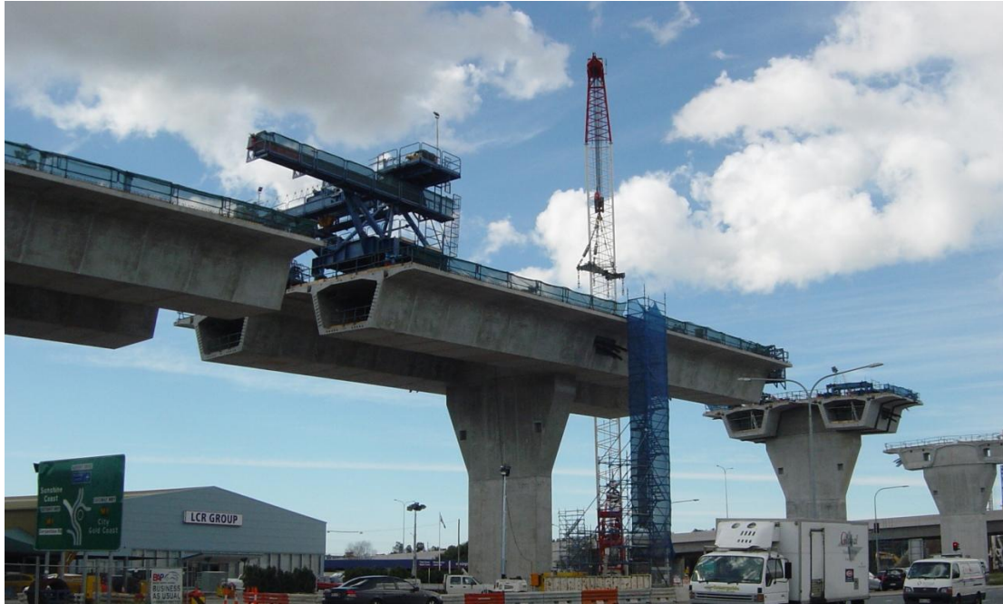
Bridge Construction (Source: CSIRO)
