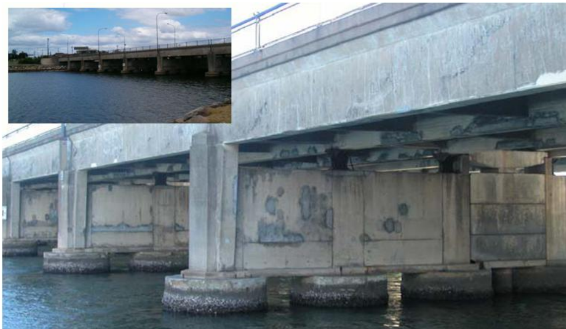
Figure 5-2 Bridge BB1 constructed in 1925 and 1959, in Sydney (Source: RTA)
